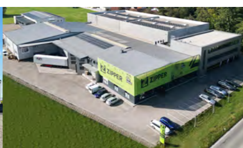
LOGISTIKZENTRUM SCHLÜSSLBERG ZIPPER-ZENTRALE
